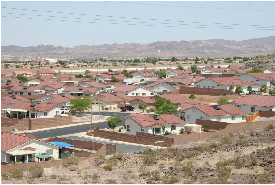
Fig. 4 Walls enclosing the backyards in this Henderson neighborhood at the base of Black Mountain. Such a scene is typical of those found in all corners of the city (Photo by author, May 2007)
