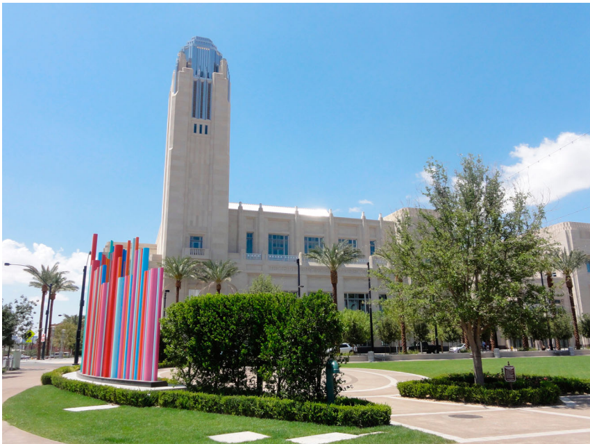
Figure 5. The Smith Center for the Performing Arts was built in an Art Deco style to evoke the era when Boulder Dam contributed to Las Vegas's growth as a tourist town. The structure is emblematic of city's diversified cultural offerings and reflects local hopes for emergence from the Great Recession. Photo by author, July 2012.
